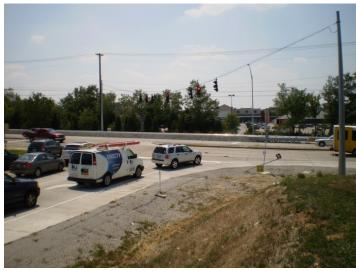
View of ramp widened at the intersection with US 31E and beginning section of concrete barrier with crash cushion (Looking west)
